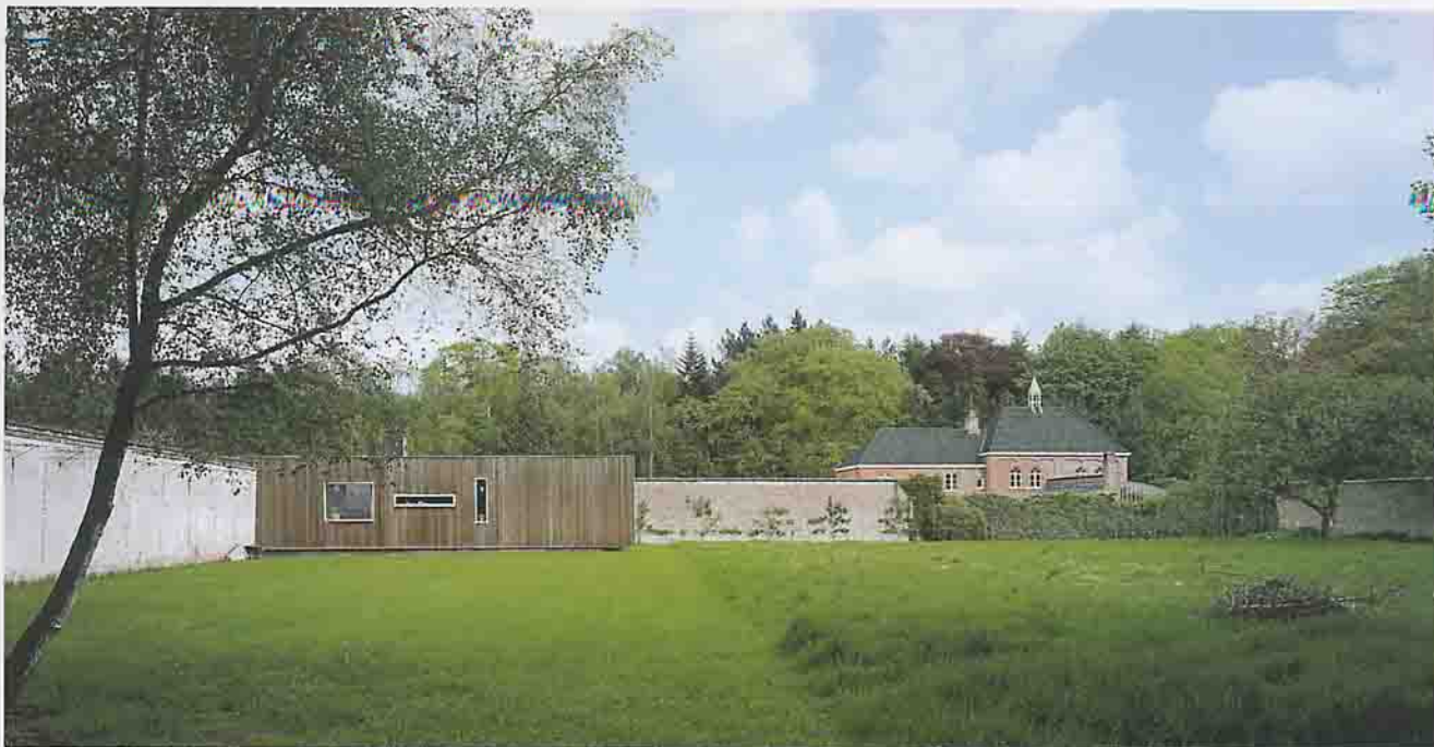
Detalle de extremo Norte de fachada Este / Detail of Northern end, East facade
